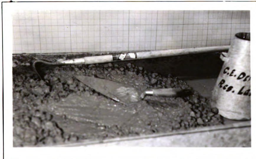
Photo shows the mix as it appeared just be- fore placing in forms
