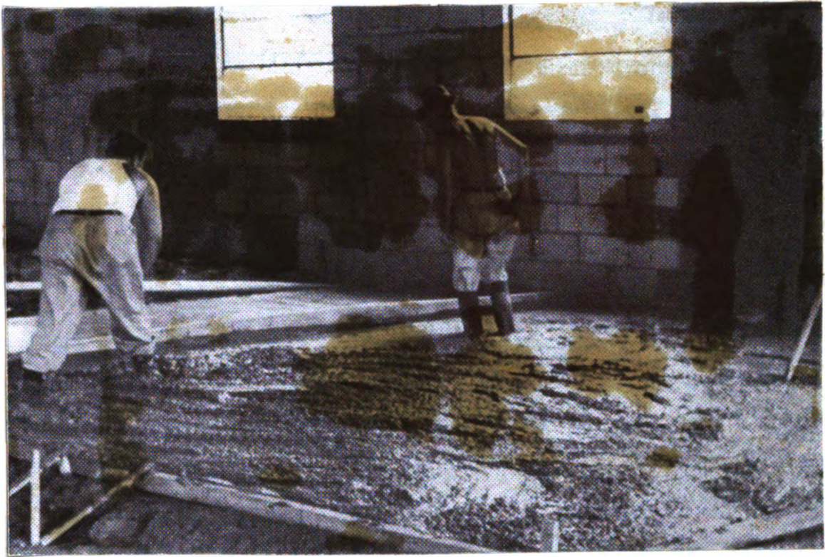
Portite-improved concrete being placed for floor of new garage to house U. S. Post Office trucks at Yonkers, N. Y.
