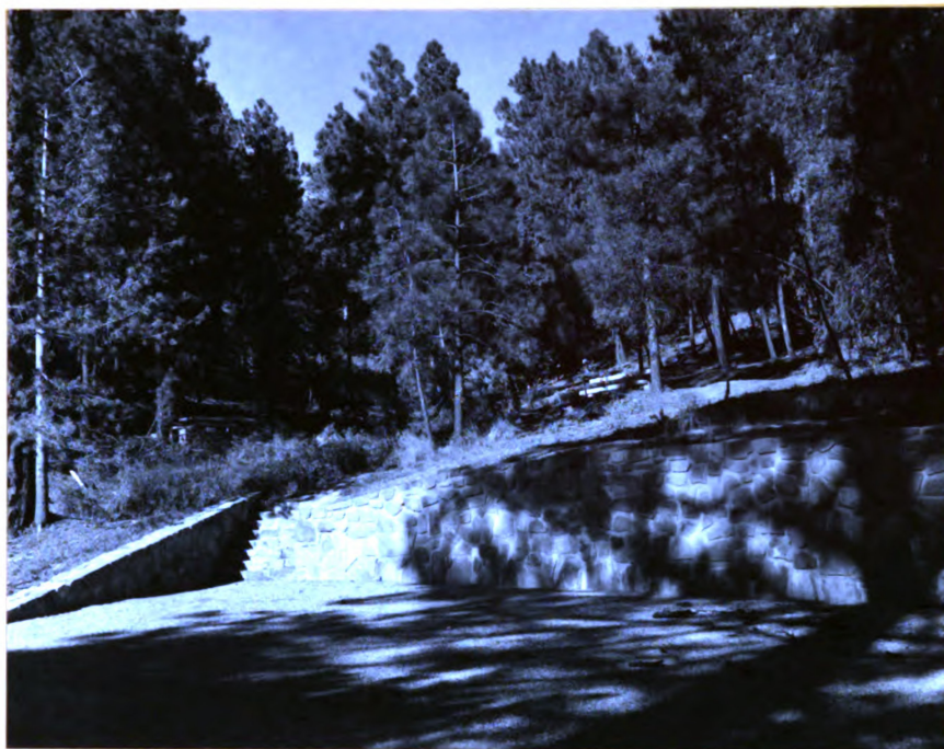
Figure 10. Retaining wall used to hold back unstable soil.
