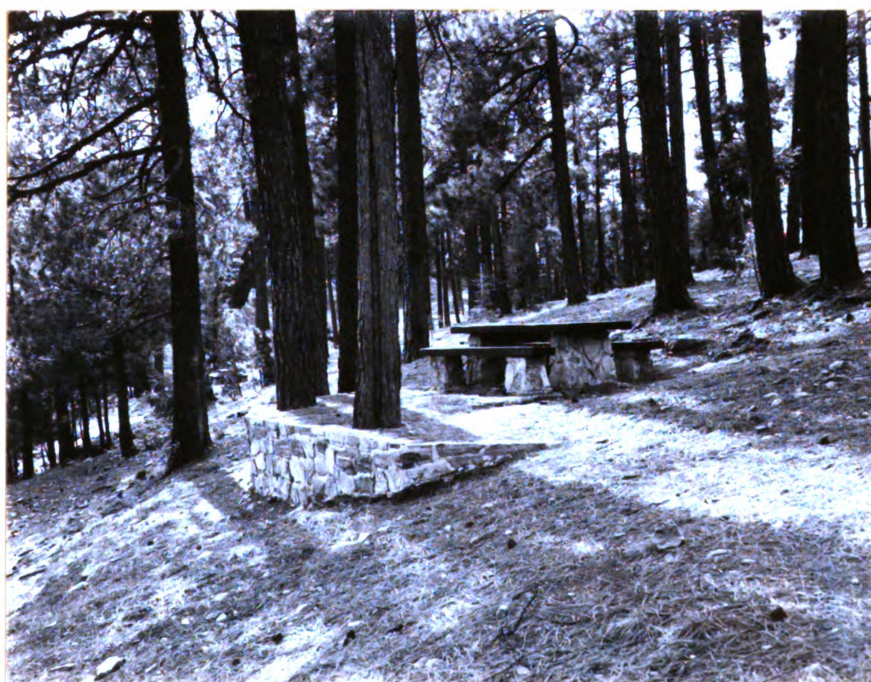
Figure 11. Masonry wall to prevent erosion at picnic sites.
