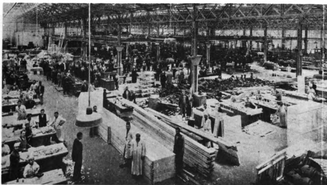
Figure 8. Misr Company for Spinning and Weaving. Wood workshop and maintenance.
