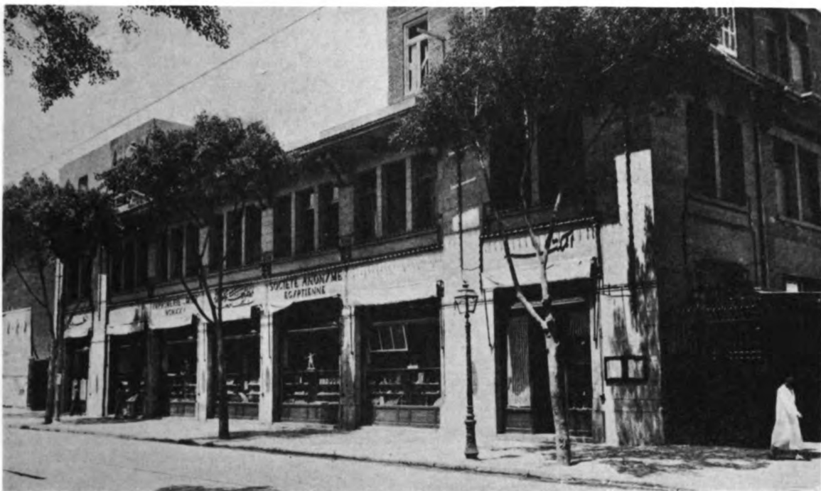
Figure 19. Misr Printing Works. Outside view.
