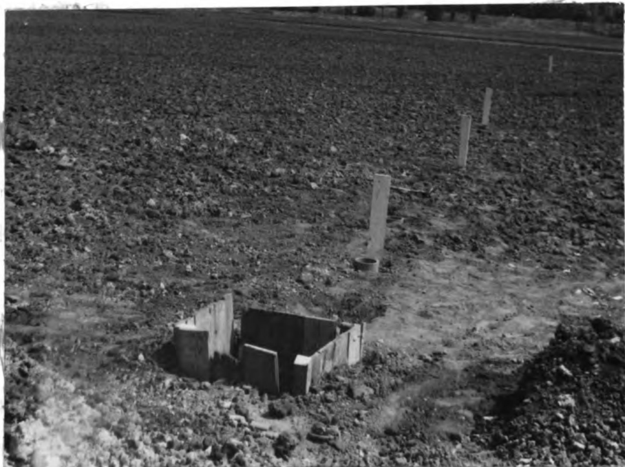
Figure 13. Sump and Observation Wells Between Tile Lines
