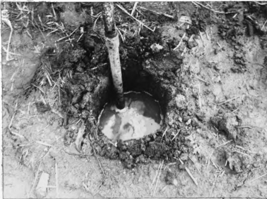
Figure 8. Uncompleted Observation Well
