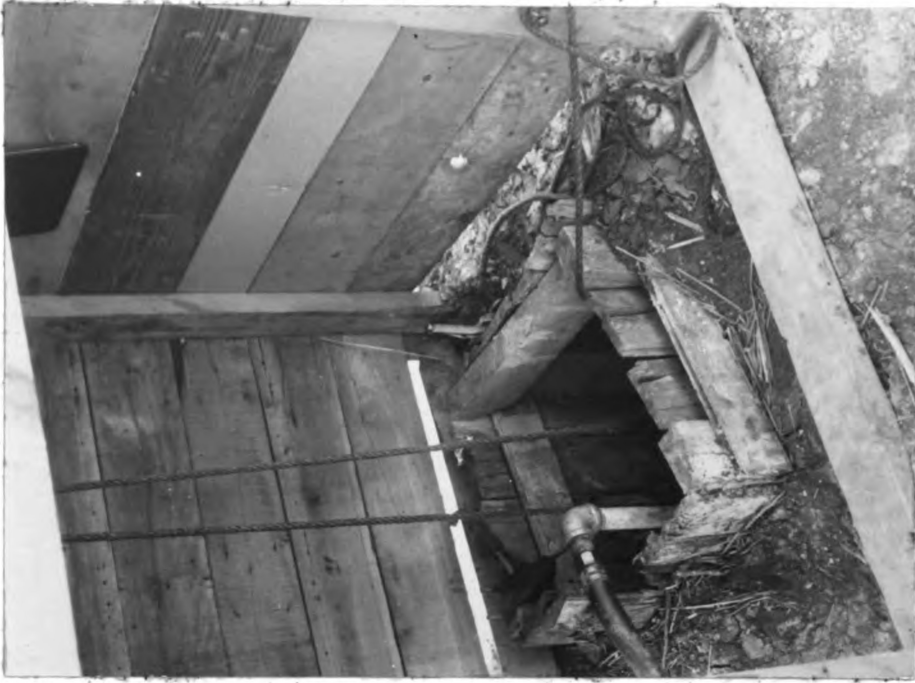
Figure 5. Sump, Showing Pump Outlet, Supporting Rope, and Sump Box
