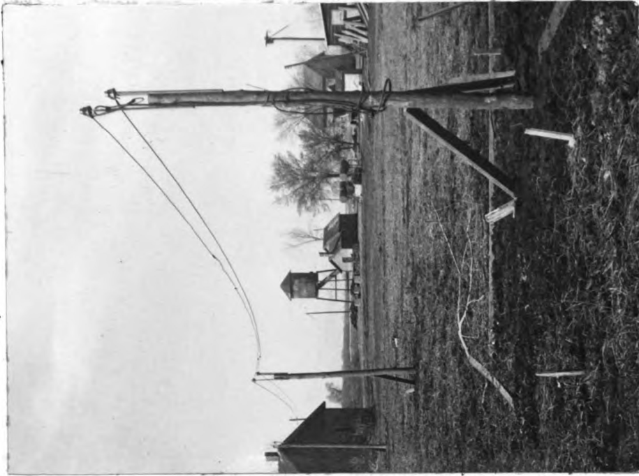
Figure 4. Electric Poles Wired to the Sump Location
