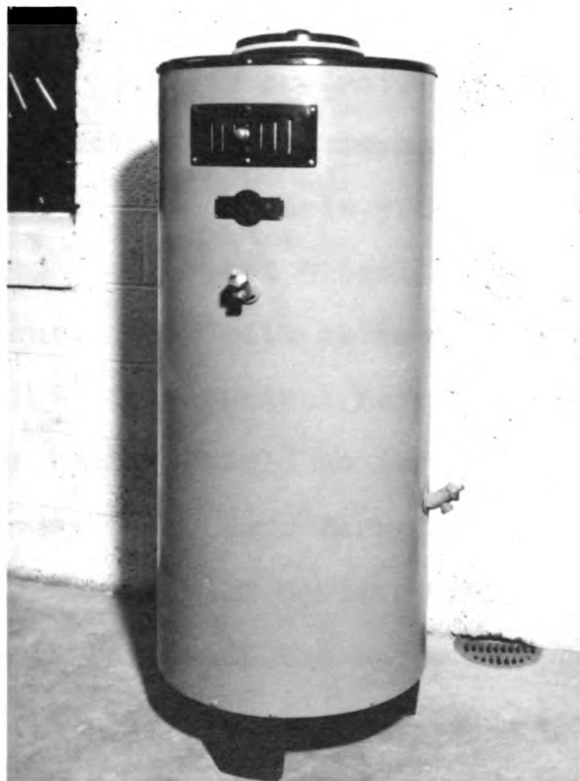
Figure 8. Combination Water And Space Heater For Use In Milk Houses.
