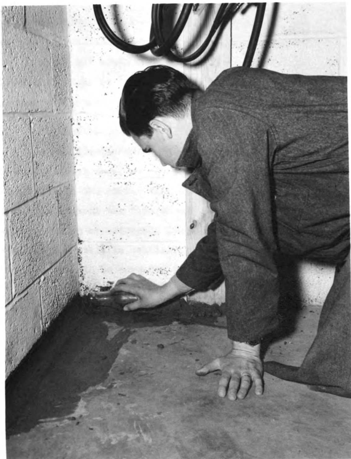
Figure 17. Construction Of The Cove Between The Walls And Floors Of Milk Houses.
