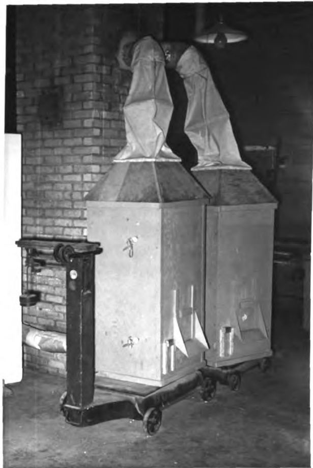
Figure 3 Bins on Scales and Exhaust System.
