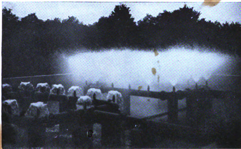
Showing Aerator Operation through Combined Altitude and Aerator Control Valve
