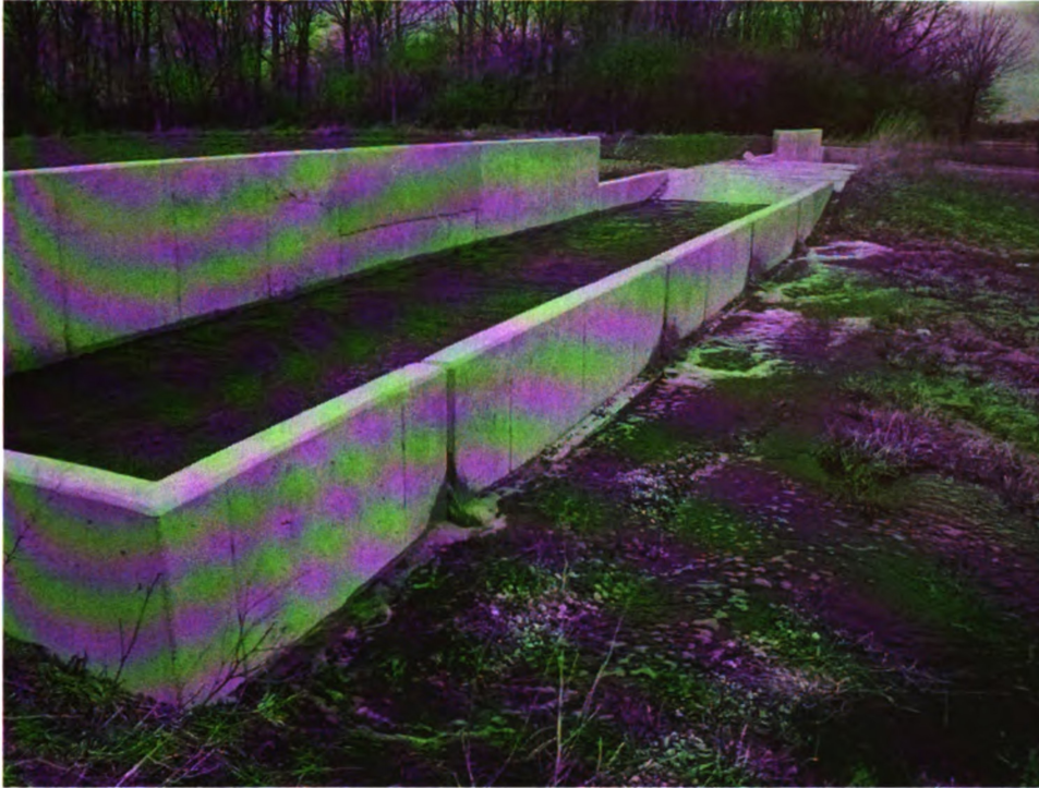
Figure 2: Filter Strip Influent Flow Dispersion
