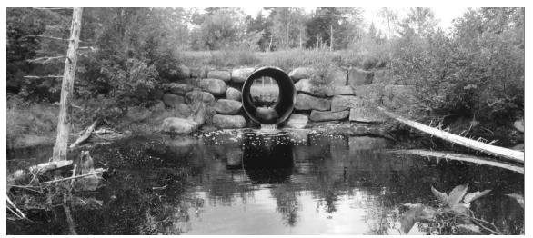
Figure 7. Traditional round culverts tend to be undersized relative to bankfull conditions and placed above the streambed, causing fish passage barriers during some or all flows and altering/fragmenting natural flow regimes and stream processes (photo by K.Mueller).
