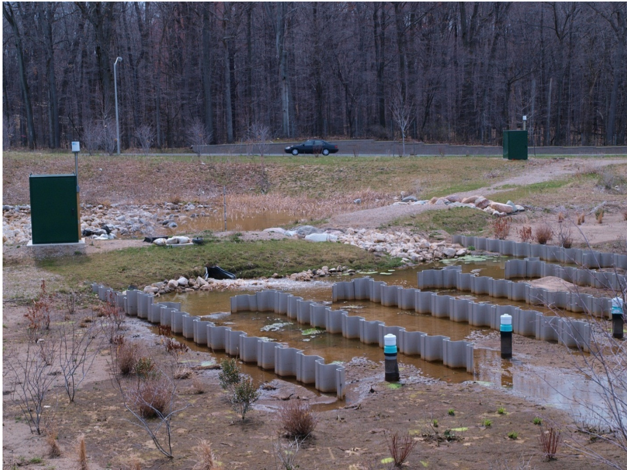
Figure 9 View of Farm Lane Bioretention Basin, from Left to Right, Equalization Basin, Influent Sampler, Ponded Area, 5 Research Cells, Main Bioretention Basin, Effluent Sampler, Service Road is Shown in the Background
