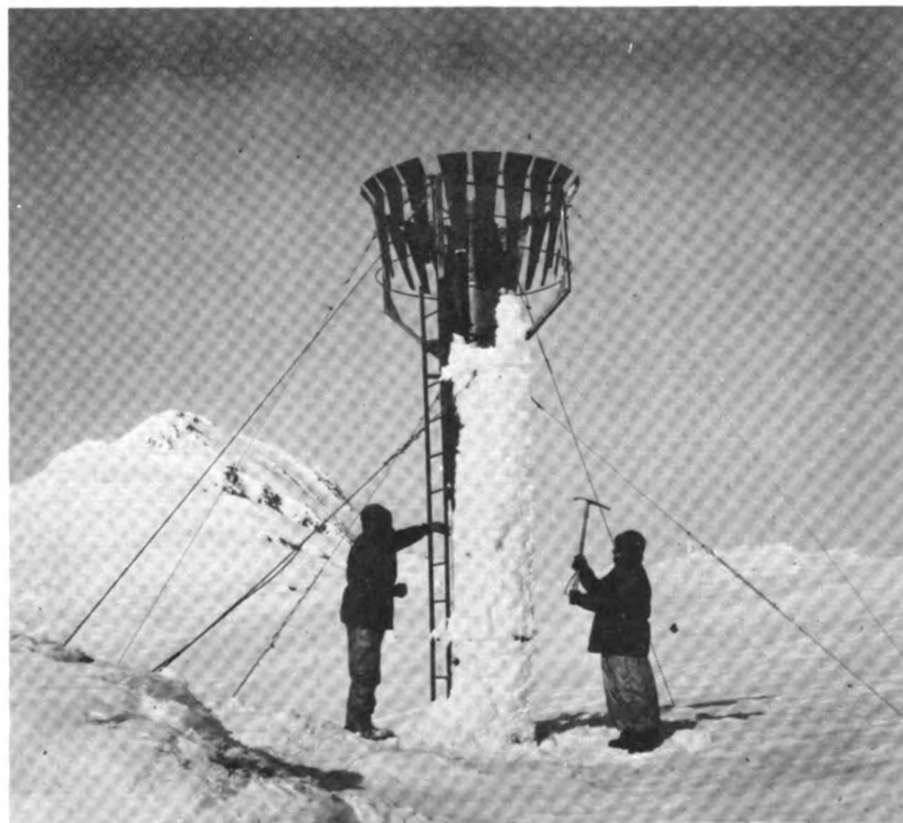
FIG. 3D.--Storage Precipitation Gage (on Lemon-Ptarmigan Ridge ) near Camp 17 (Photograph by M. M. Miller).
