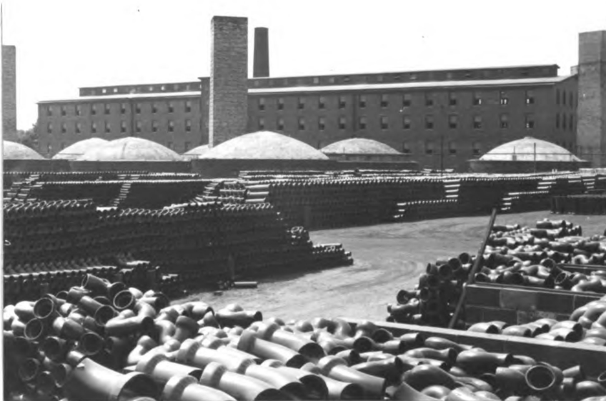
Figure 22. American Vitritified Tile Company. Dome-shaped structures are bee-hive kilns.
