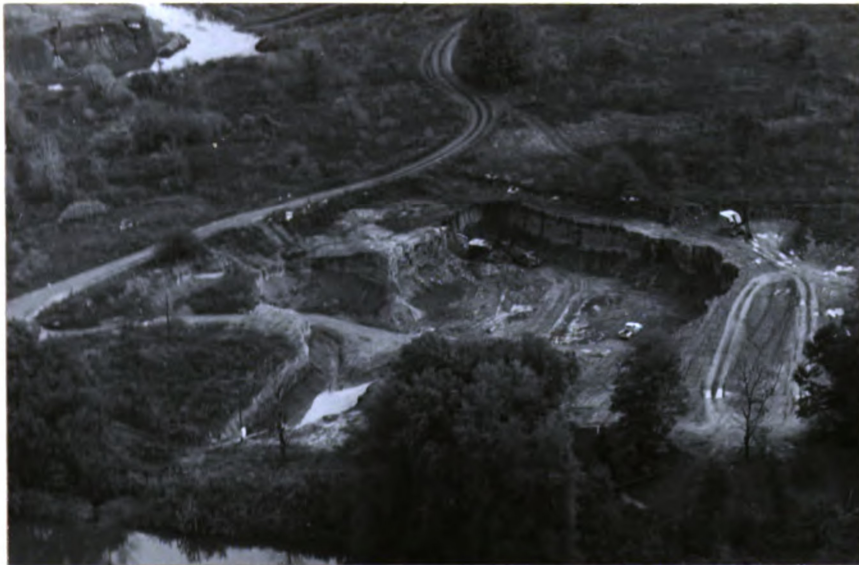
Figure 24. Air view looking northeast of mine presently used by Grand Ledge Clay Products Company. Steam shovel to the right of the pit is clearing away overburden. Note proximity of river and size of equipment in relation to depth of pit.
