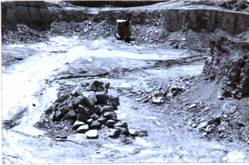
Figure 23. Active clay pit of the American Vitrified Tile Company located just outside the Grand Ledge city limits. Note size of steam shovel in relation to depth of pit.
