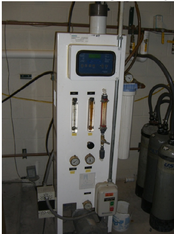
Figure 12: The reverse osmosis unit is activated when the reservoir drops to a set level
