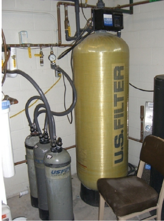
Figure 11: Tempered water is softened and passed through carbon filtration.
