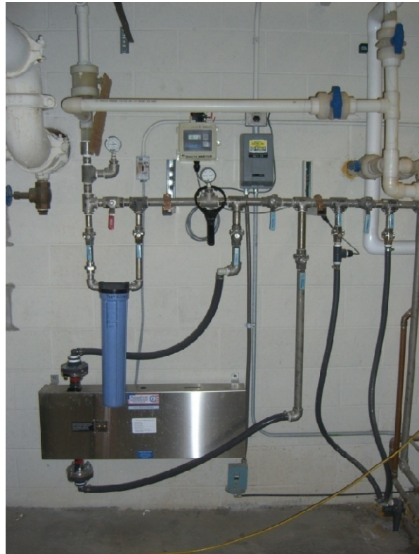
Figure 14: Before water is circulated through the building, it is passed through an ion-exchange resin, a 22 \mu\text{m} filter and a fluorescent lamp.
