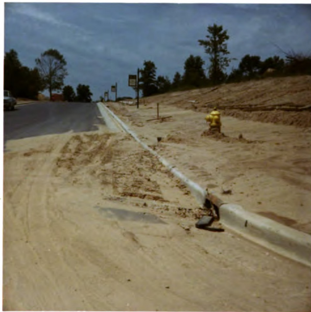
Figure 12.--Sediment damages streets and storm drains. Over eighty per cent of all material eroded from construction sites was initially deposited in streets and storm drains. Its removal becomes a social cost.
