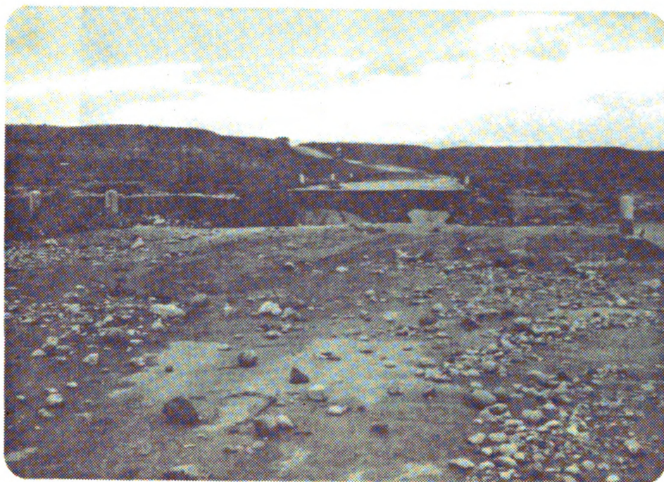
Figure 4. A road washed away by run off in a wādī (near Bir-Ganam).
