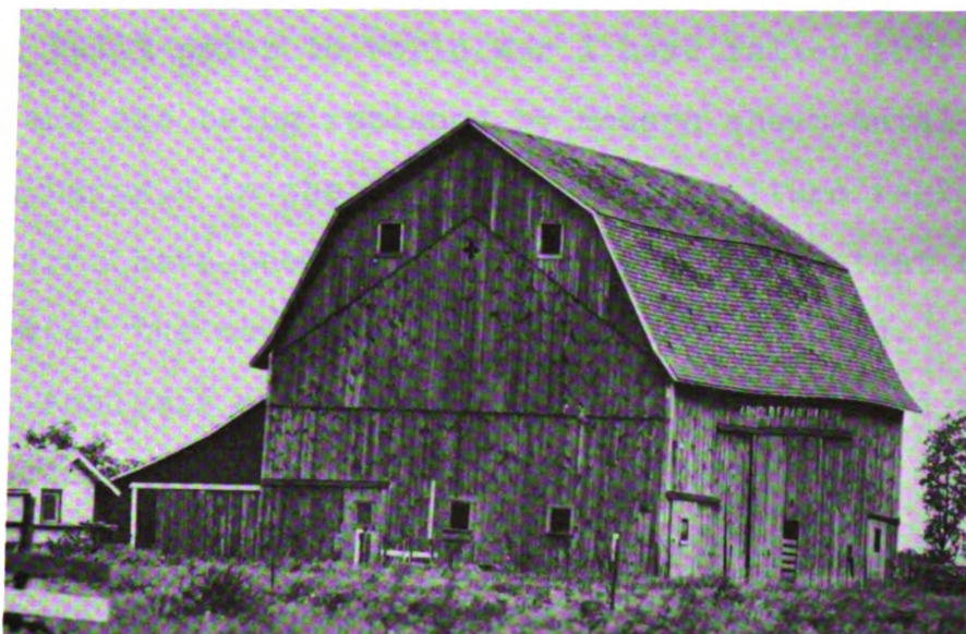
Figure 27: -- New England barn modified to increase hay storage capacity by addition of a gambrel roof. The modification here is clearly visible at the old gable-roof line.
