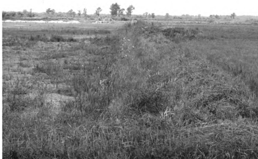
Fig. 45. -- A dike at Central, constructed about seventy years ago. It is too narrow for machinery, and will be replaced.
