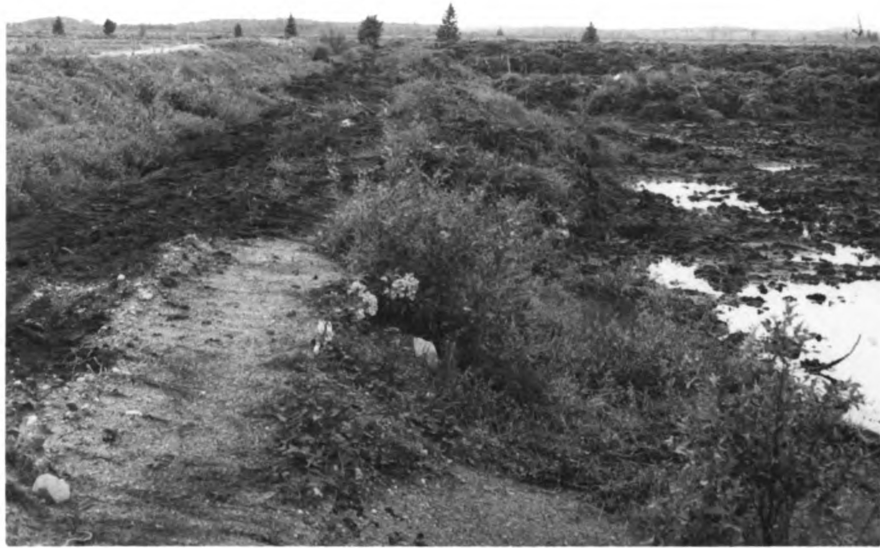
Fig. 40. -- Bog construction at Thunder Lake, North-central region. The peat soil is only partially decomposed.
