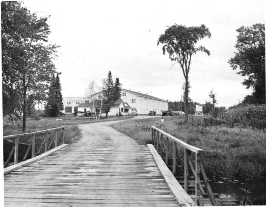
Fig. 51. -- Warehouse and other buildings at Cranberry Lake. Cement block warehouse was constructed using sand from the property. It is the largest in the state. Note weather instrument shelter.
