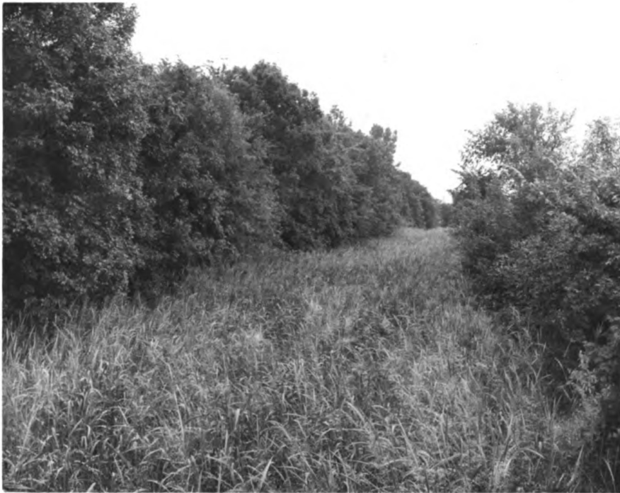
Fig. 23. -- Canal from Berlin marsh to Fox River, completely choked by grasses. The alkaline water of the Fox is chiefly responsible for the serious growth of weeds.
