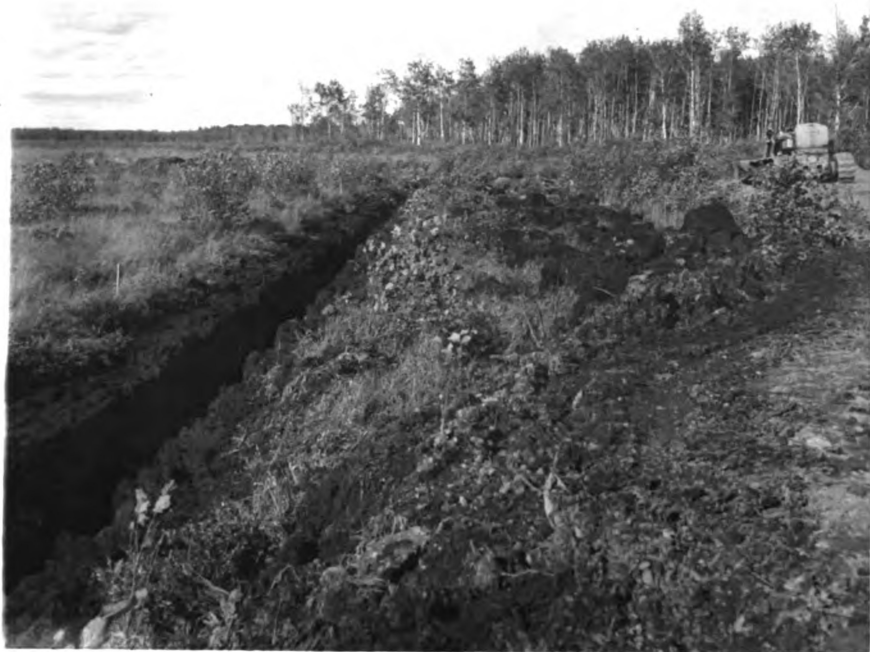
Fig. 42. -- New bog construction in the Northwestern region. The peat here is more decomposed than in the North-central region.
