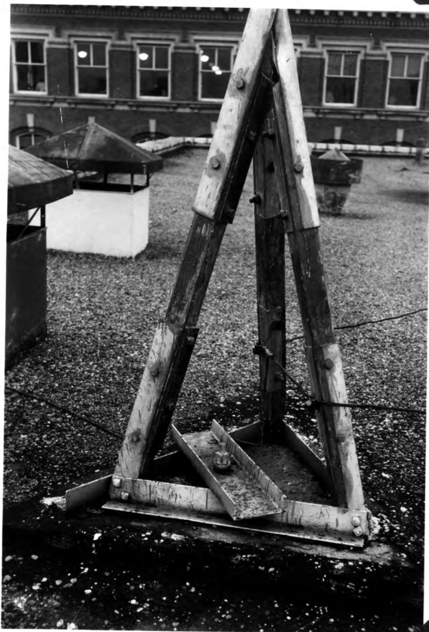
One tower leg insulator October 29, 1935. Entire tower built by WKAR staff.
