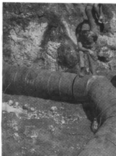
Fig. 36. Sewer line of welded empty gas drums.
