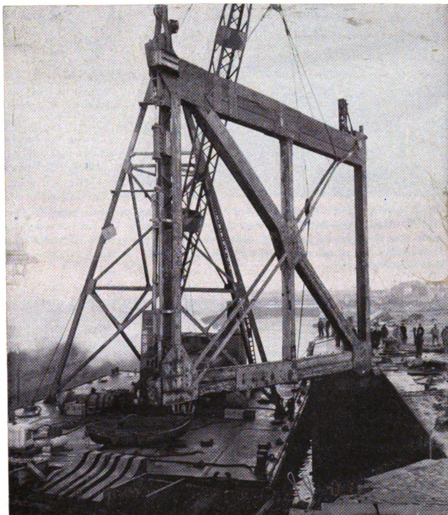
Fig. 11. Installing a gate strut.
