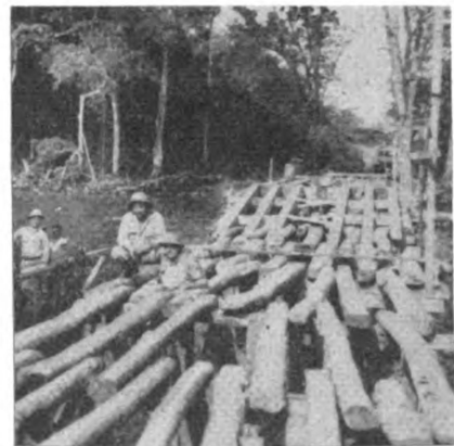
Fig. 29. Timber bridge under construction.
