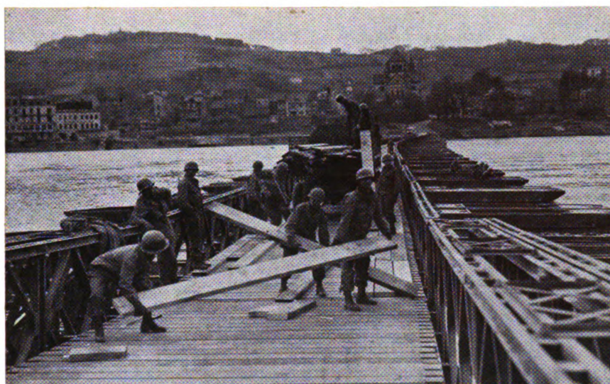
Fig. 22. Floating Bailey bridge.
