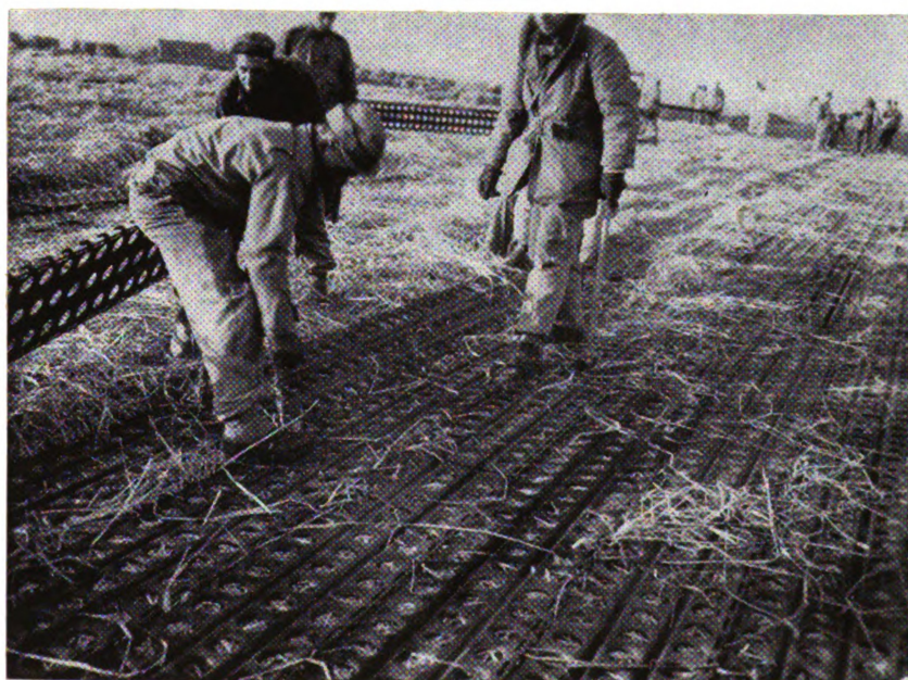
Fig. 25. Laying pierced steel plank.
