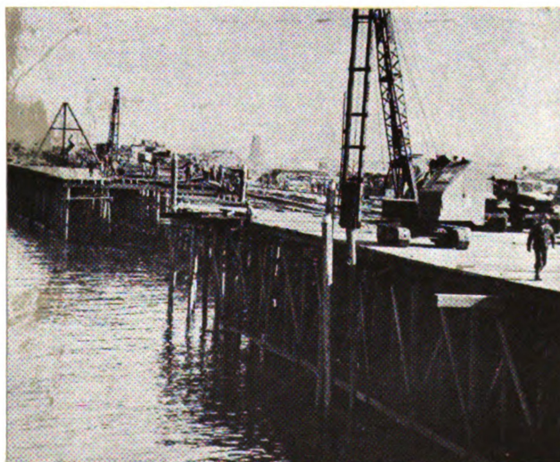
Fig. 4. Driving piles for wharf decking.
