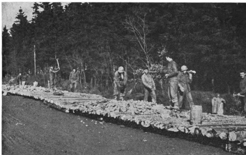
Fig. 10. Corduroying as an alternate method.
