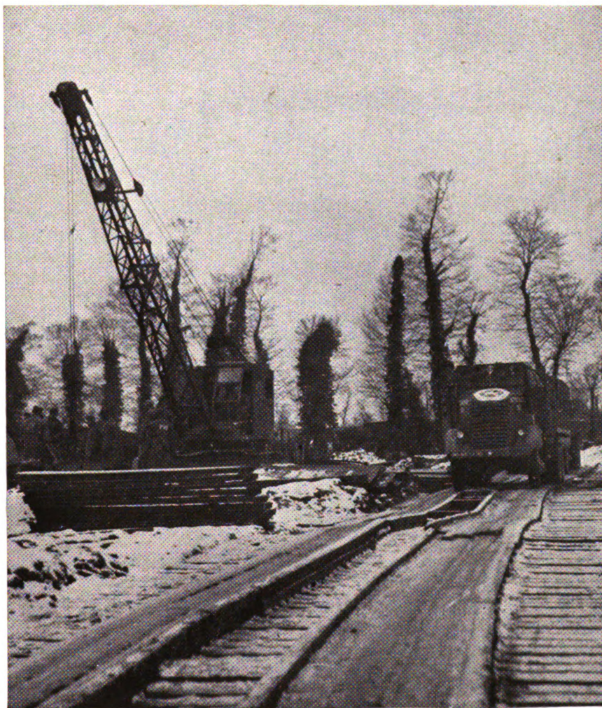
Fig. 9. Timber plank road.
