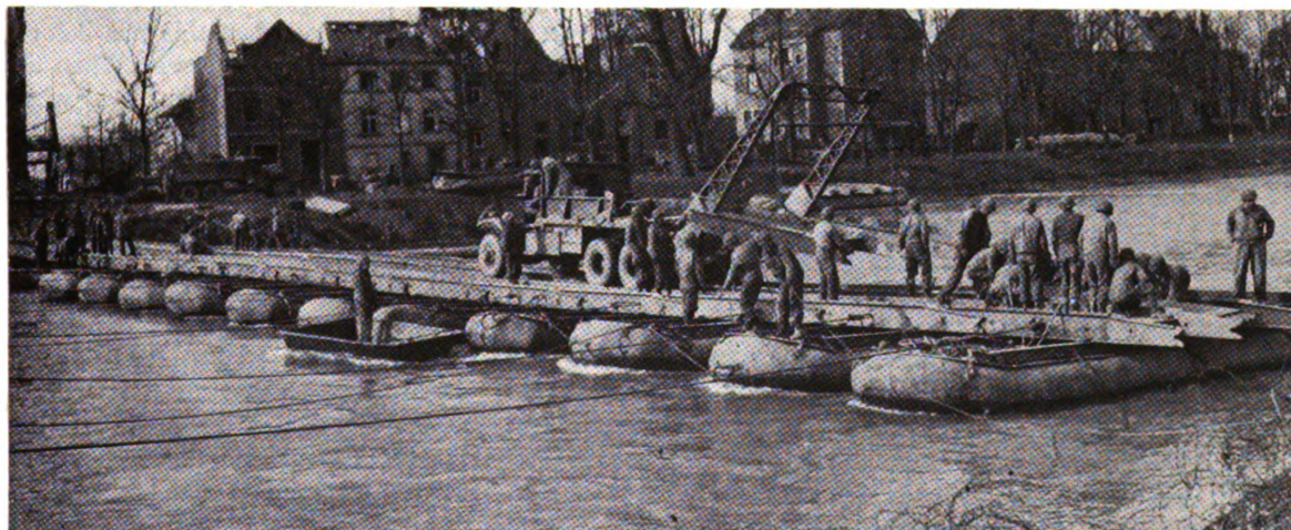
Fig. 23. Floating treadway bridge.
