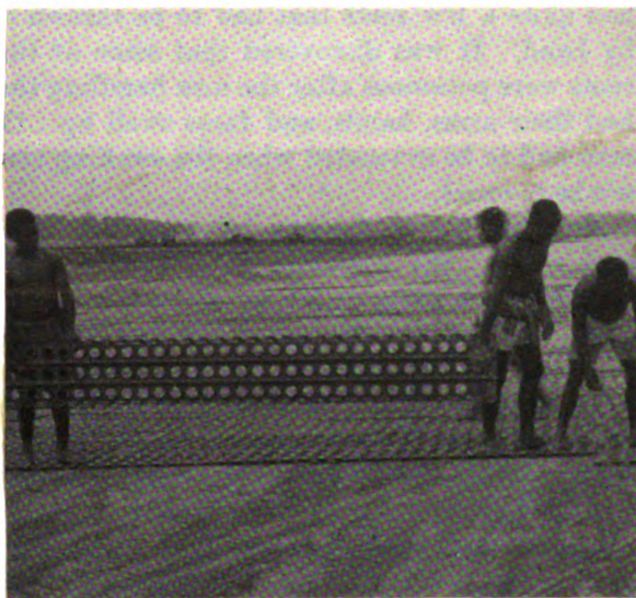
Fig. 34. Laying pierced steel plank.
