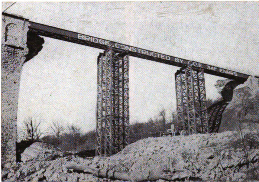
Fig. 13. Railroad bridge of meter beams.
