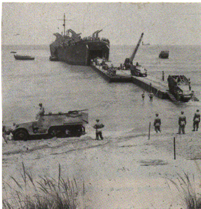
Fig. 28. Pier formed by momentum beaching.
