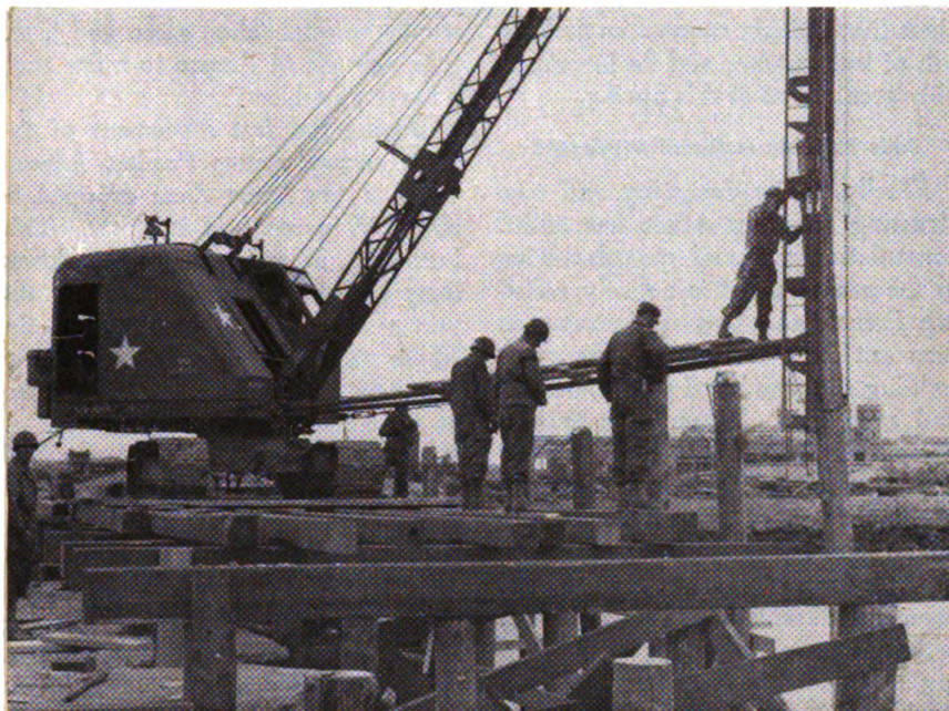
Fig. 5. Engineer's pile driver in action.
