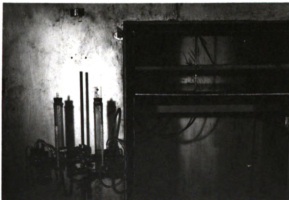
Fig. 3 Soil moisture control system
