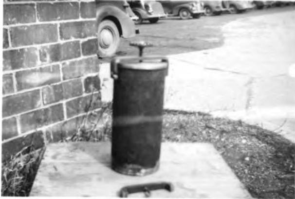
The apparatus for determining the air content of concrete is shown above.
