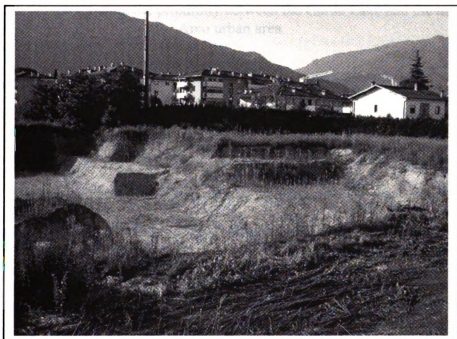
Figure 5.7: image showing the Arco School construction site.
