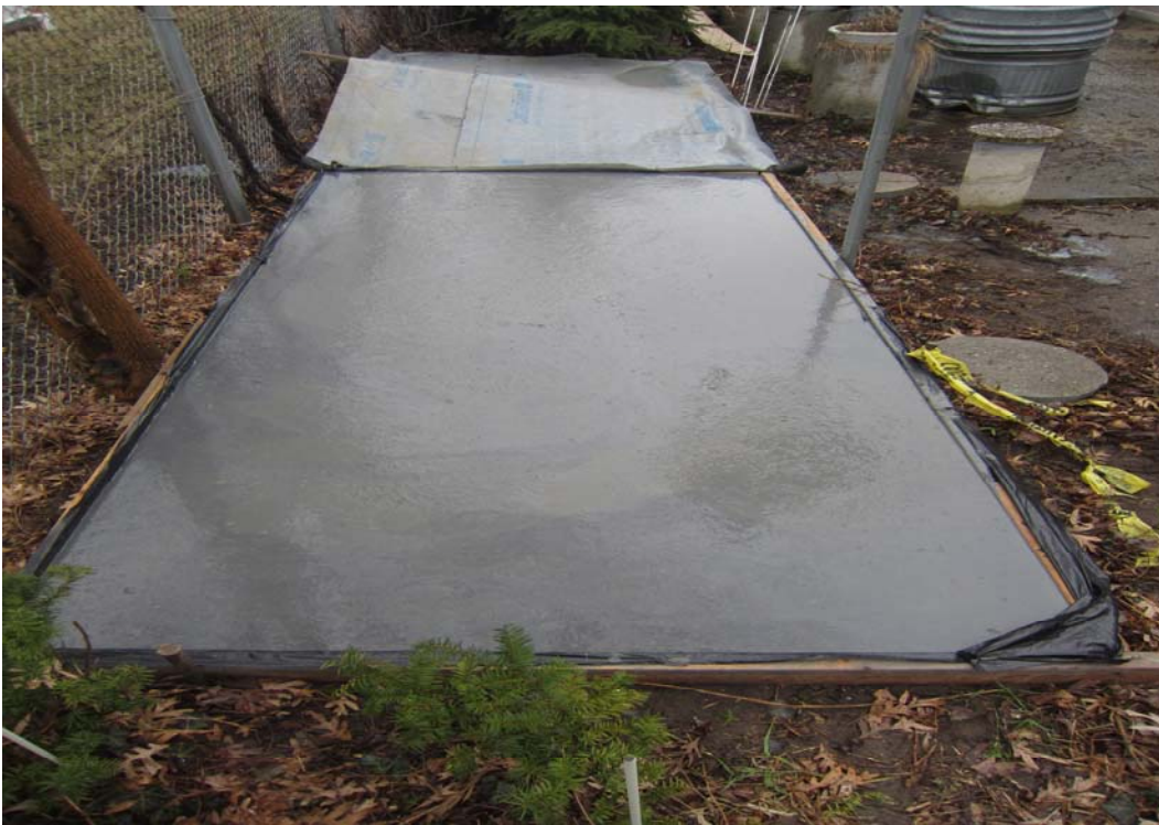
(d) Overlay outlook of high-strength concrete after being laid
