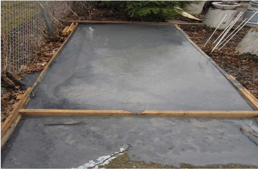
(c) Overlay outlook of high-strength concrete after being laid
