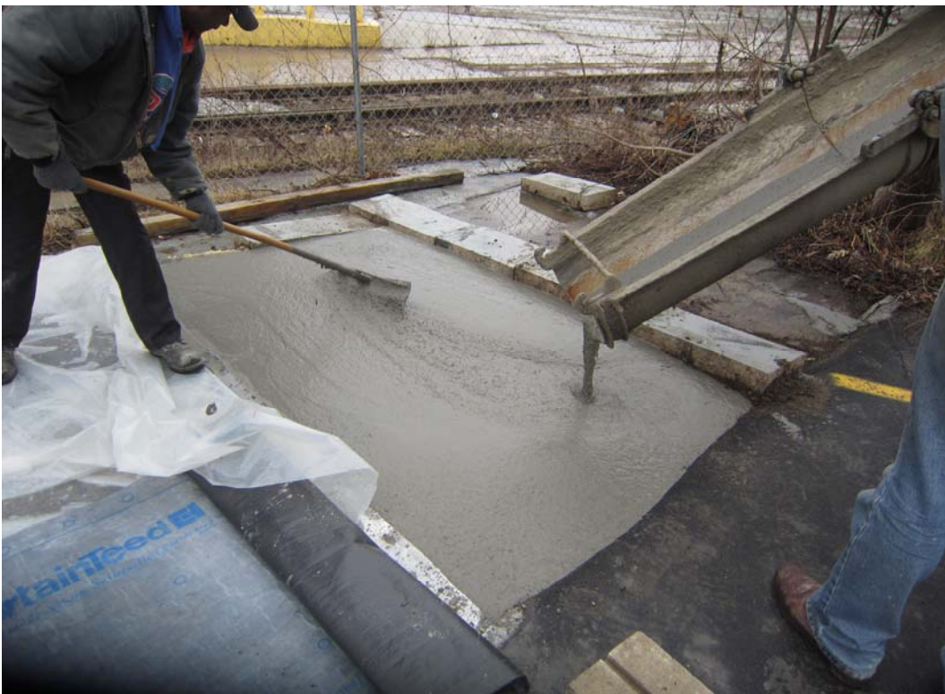
(b) Pouring of concrete for slab
