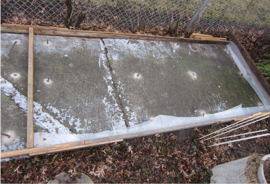
(a) Preparation of old slab for an overlay
