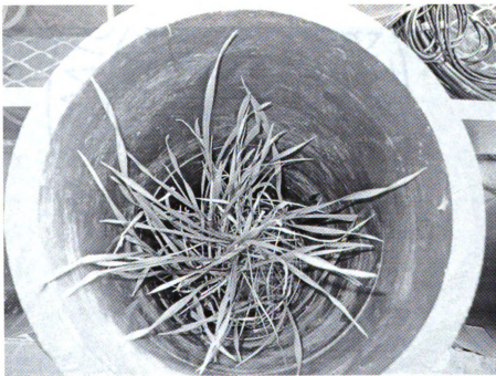
Figure C14: View into column after rain event.
