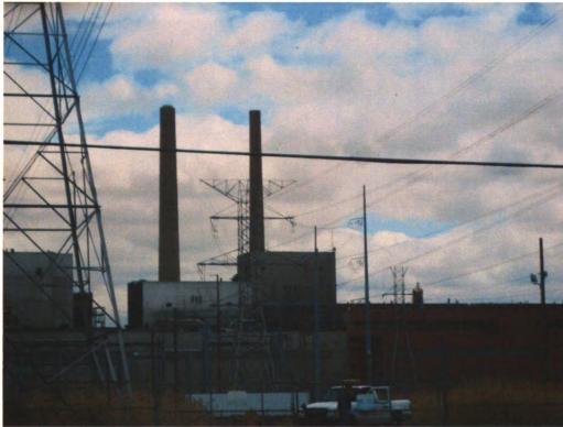
Figure 1.4: Detroit Edison's St. Clair power plant. Photo by author (2009).
