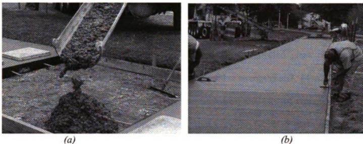
Figure 6.2 Construction of the sidewalk/maintenance vehicle pavement with recycled glass concrete (a) pouring of concrete; (b) finishing of concrete
