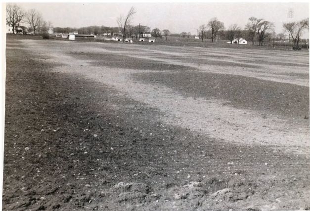
Figure 13. View over the South Field at the Farm Crops Farm looking northwest. Notice how the tile lines affect the field drainage pattern.
