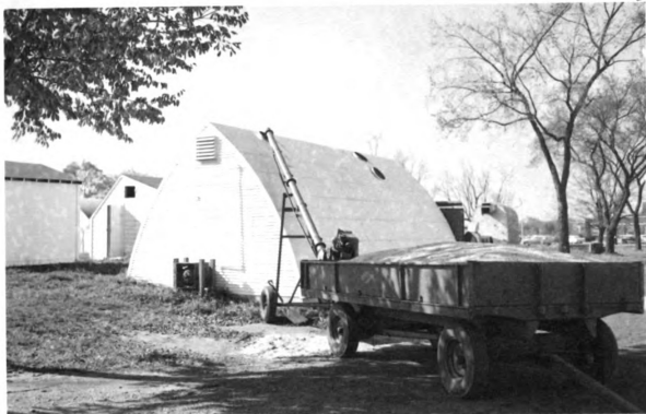
Fig. 1a. Filling the bin with shelled corn through hatch openings
