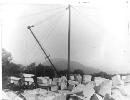
Fig. 21.--Boom-derrick in operation at West Rutland marble mine-quarry.
