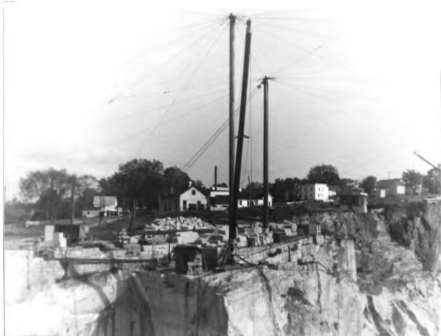
Fig. 18.--Multiple boom-derricks used in a Rock of Ages Corporation granite quarry in Graniteville.
