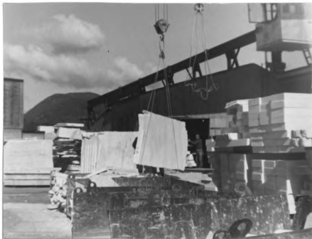
Fig. 23.--Overhead crane at Green Mountain Marble Company's finishing mill in West Rutland.
