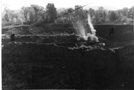
Fig. 26.--Blasting slate beds loose from the quarry face near North Poultney.
