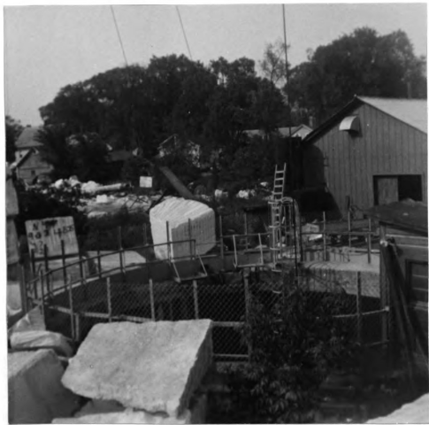
Fig. 19.--Vertical-shaft entry of marble mine-quarry at West Rutland.
