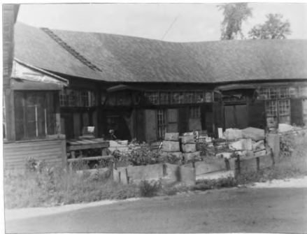
Fig. 22.--Circular granite shed built to accommodate stationary derricks.
