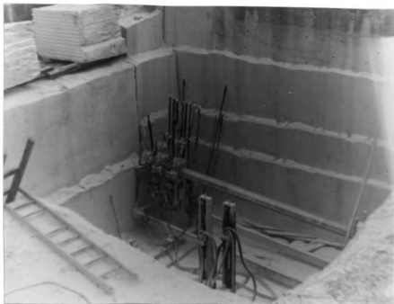
Fig. 20.--Channelbar being used in new marble mine-quarry at South Dorset.
