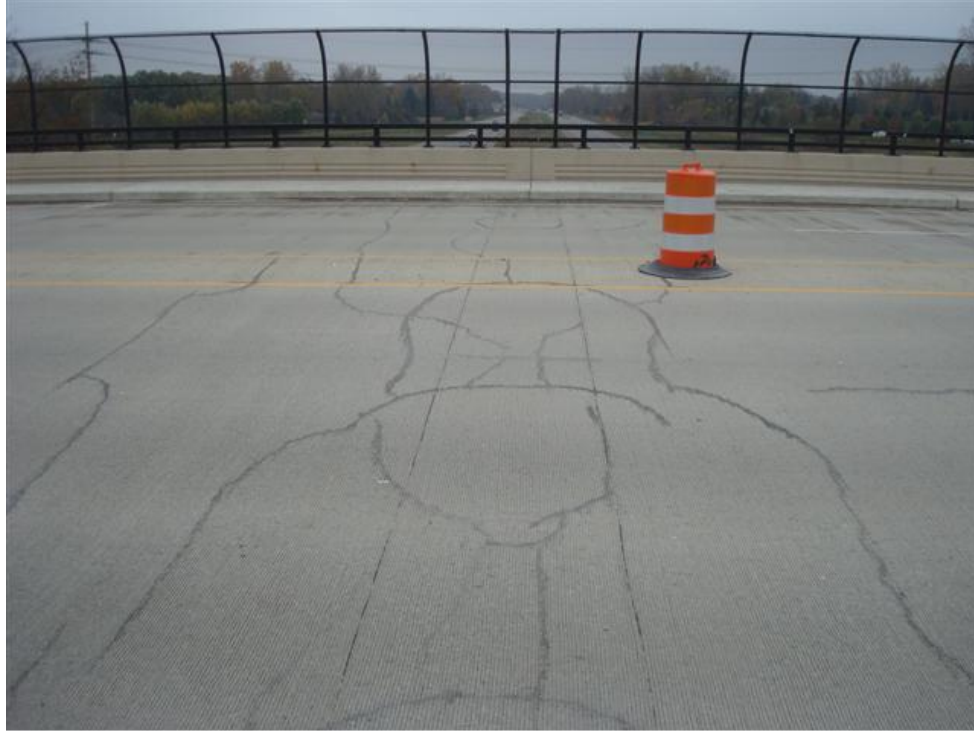
Figure 12. Transverse cracking over pier/negative moment region (Bridge No. 13, 26 mile Rd. over M-53)
