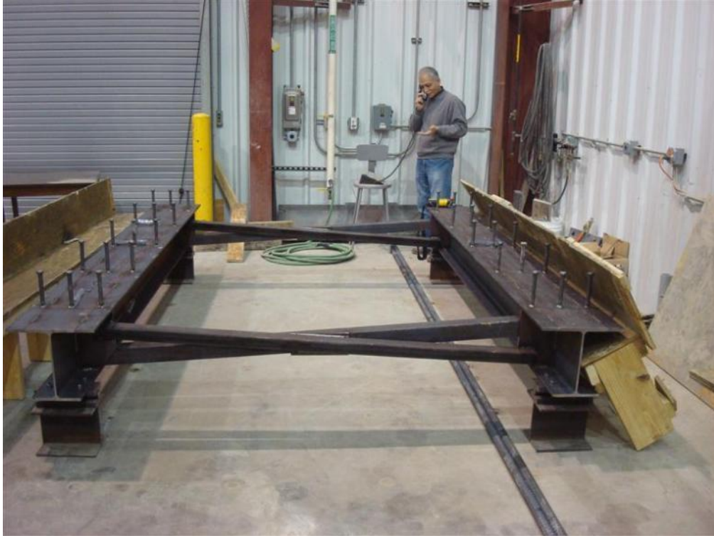
Figure 39. Test Unit 3 Steel Frame Assembly
