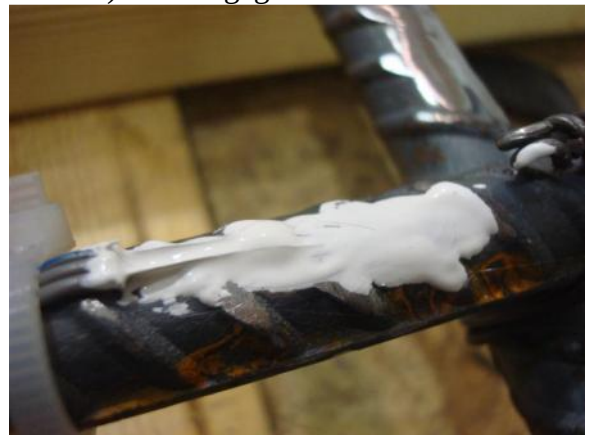
d) Assembly covered with M-Coat D
