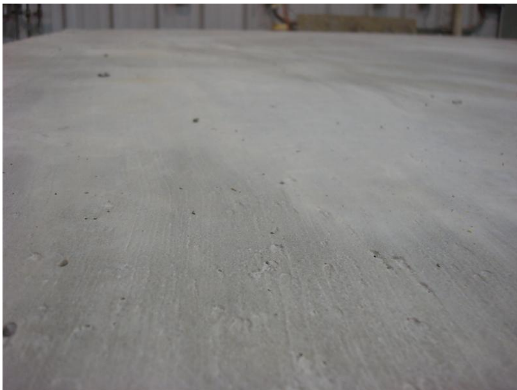
Figure 58. Close-up of completed test unit top surface (test unit 4)
