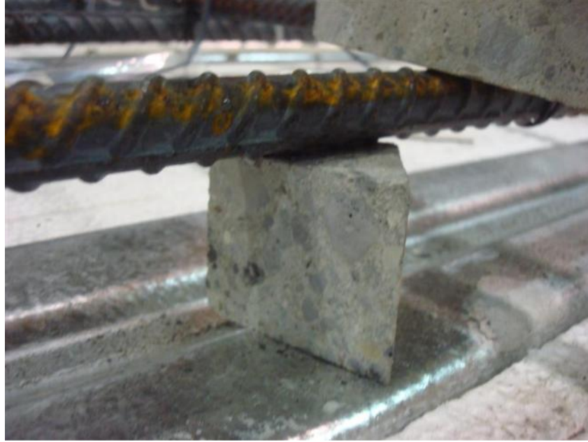
Figure 47. Concrete spacers for reinforcing steel (typical)
