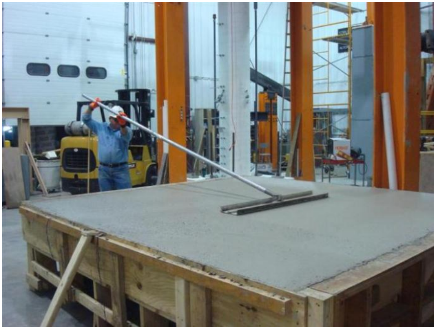
Figure 54. Bull floating the concrete surface (test unit 3)
