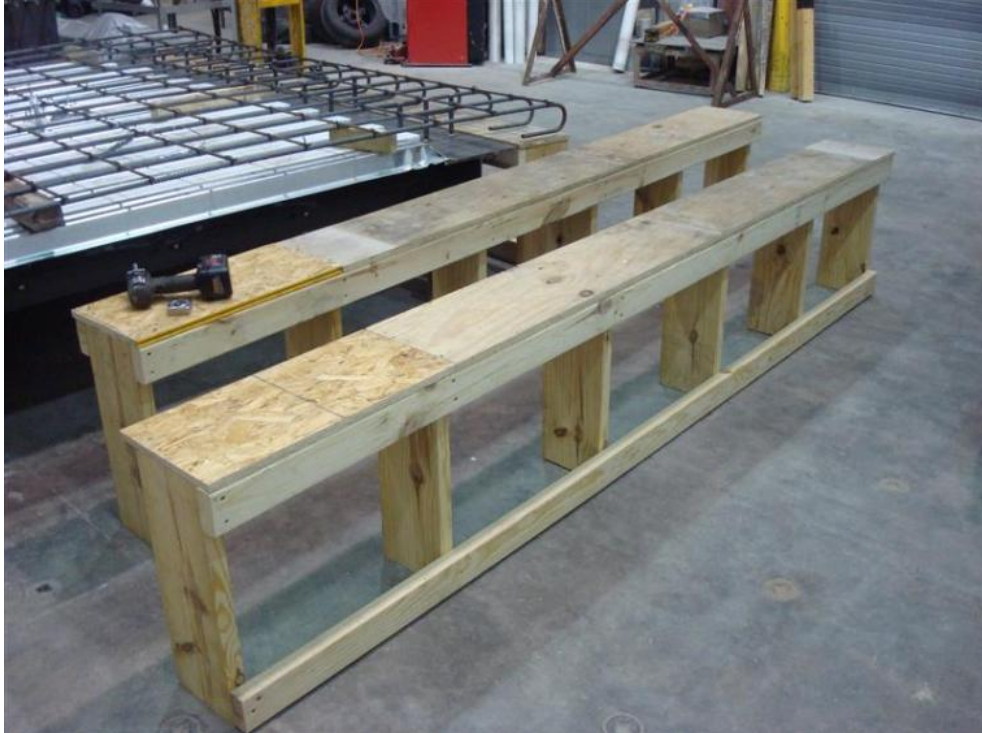
Figure 44. Cantilever forms bottom section
