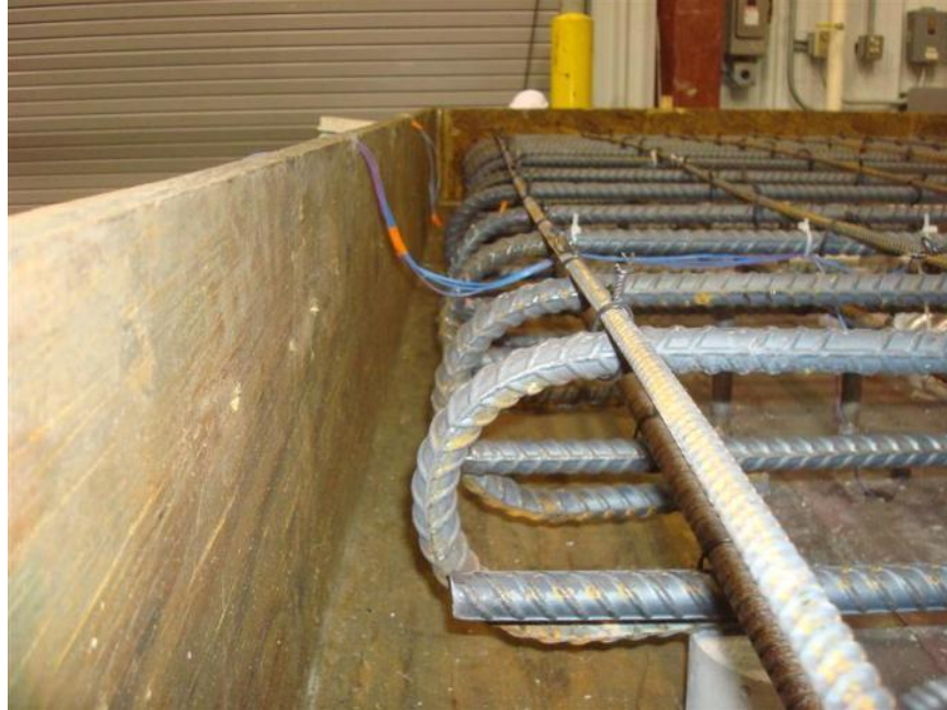
Figure 49. Reinforcing steel side cover (typical)
