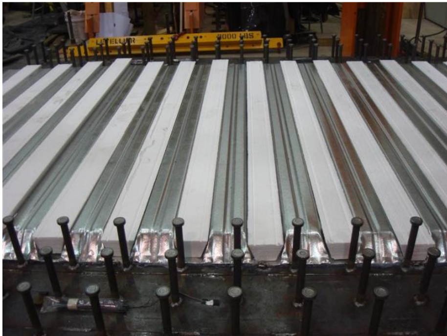
Figure 41. SIP forms Styrofoam fillers
