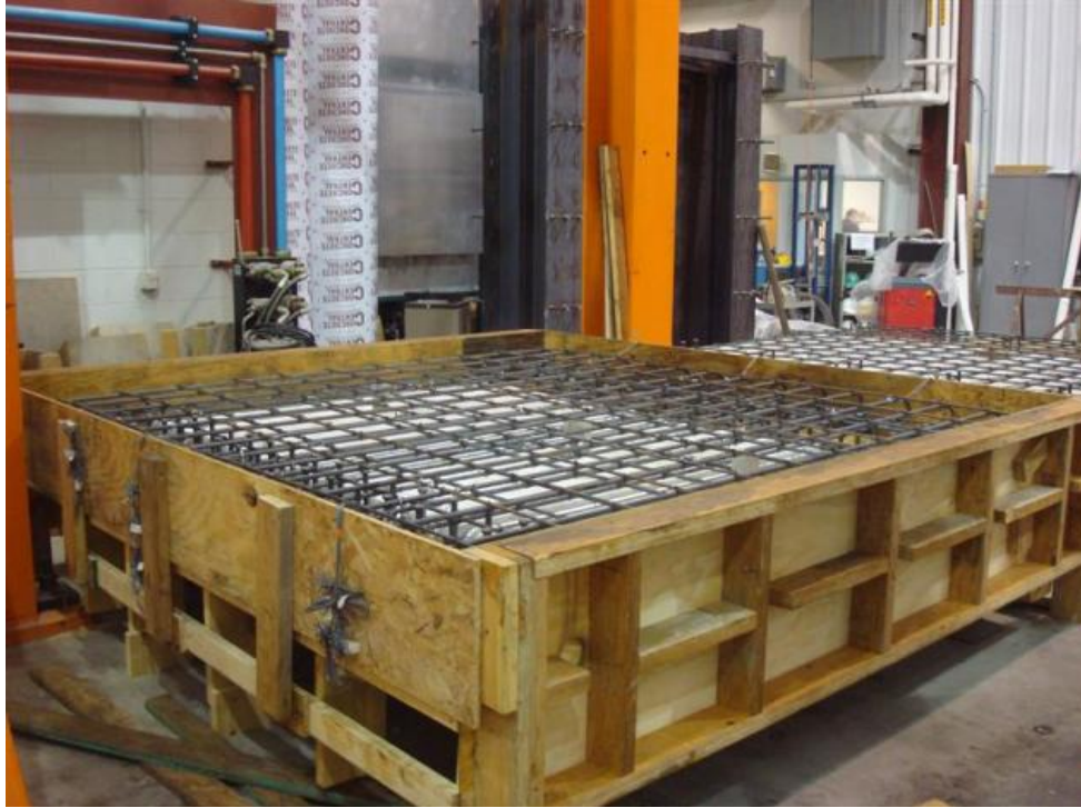
Figure 46. Completed formwork (all lumber forms are removable)
