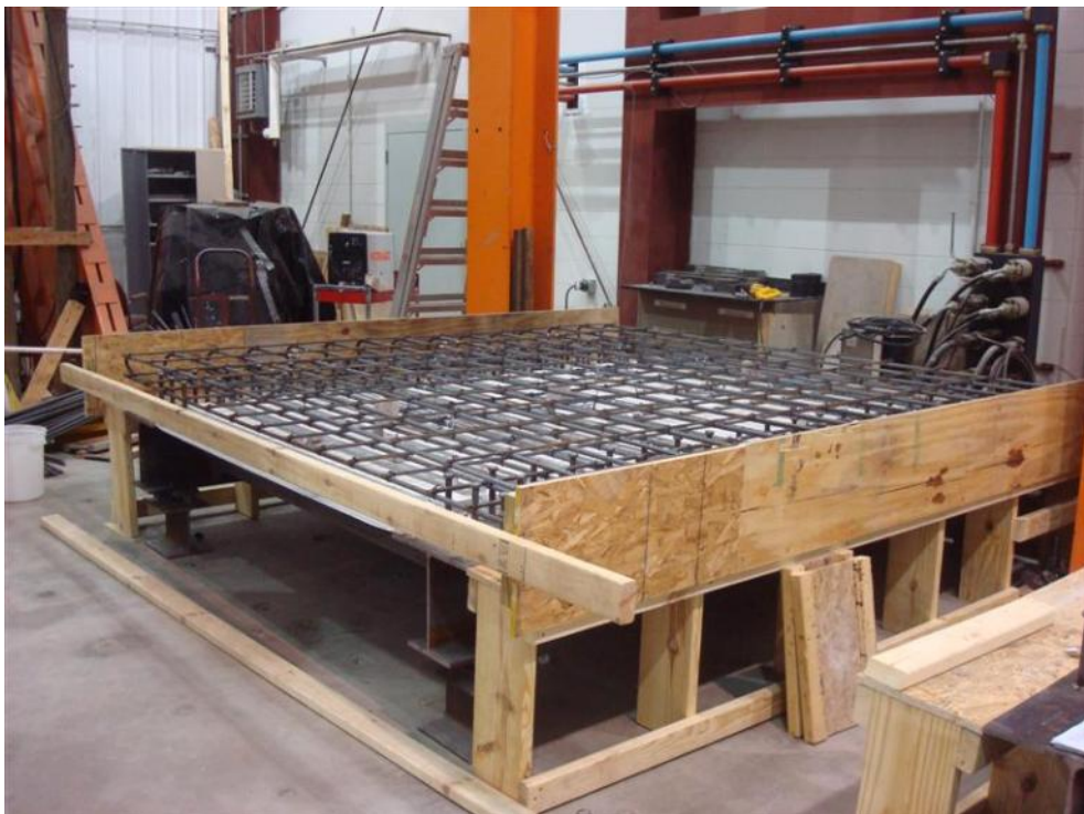
Figure 45. Completed cantilever forms
