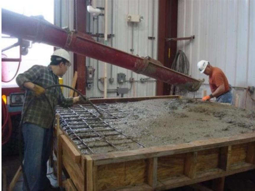
Figure 53. Placing and vibrating the concrete (test unit 3)
