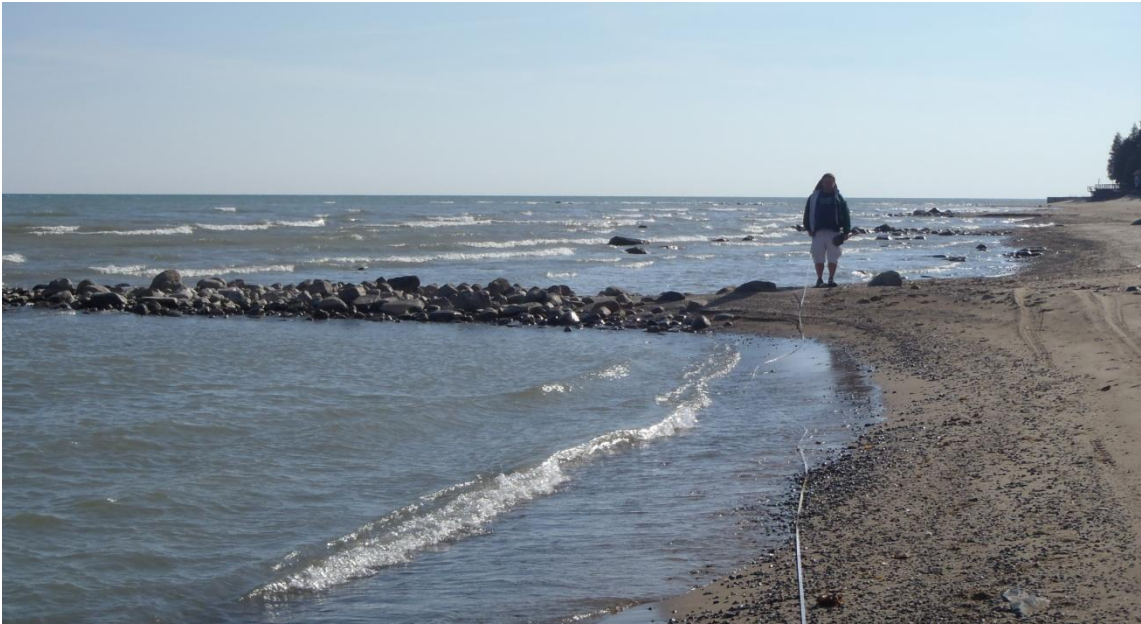
Figure 6.10: Looking south at a groin at the Sanilac County site. Note the scale of each of the three control structures present in this photograph. (photo by Phil Wernette)
