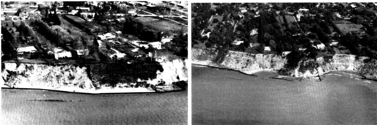
Figure 1.7: Property damage due to bluff erosion in Berrien County, MI during high lake-levels. (from Buckler and Winters, 1983, pg. 102)
