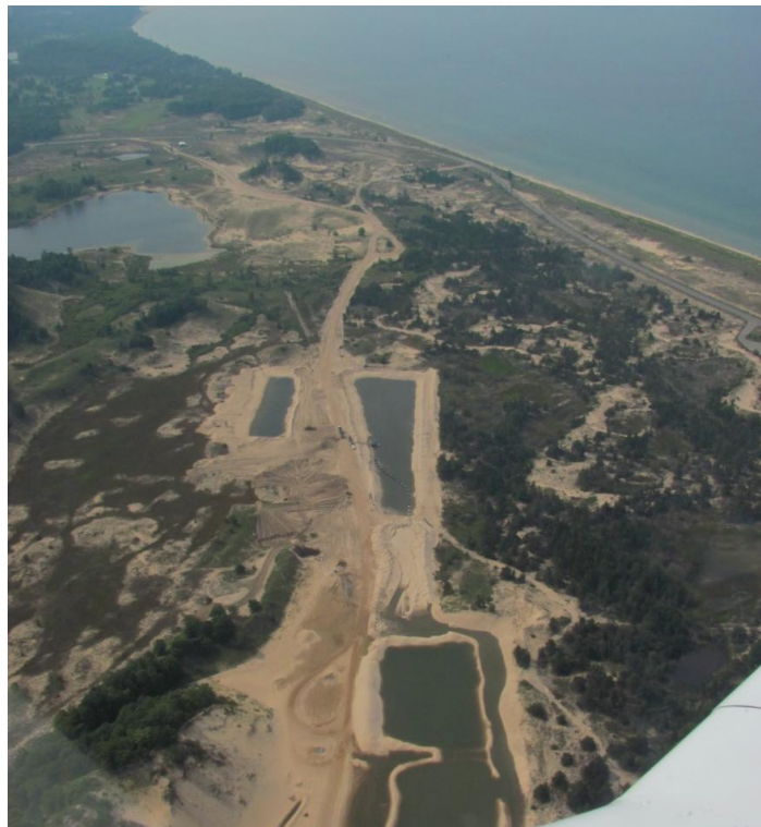
Figure 1.4: Looking south at an active sand mine in Ludington, MI. This mine, owned and operated by Sargent Sand Co, Inc., has been active off and on since 1937. Note the large rectangular ponds present where large barrier dunes were once present. (photo courtesy of Ludington State Park)
