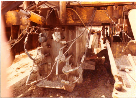
Figure 2.4. Vibrators for the Aukerman form.
