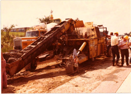
Figure 2.3. Fresh concrete being augered into the Aukerman form.
