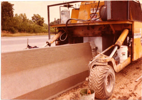
Figure 1.1. Fresh concrete structure emerging from the slipform machine.
