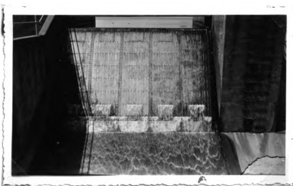
Downstream view of single gate showing minute flow trickling over. As can be seen in the picture at the top, very little leakage gets through these gates.
