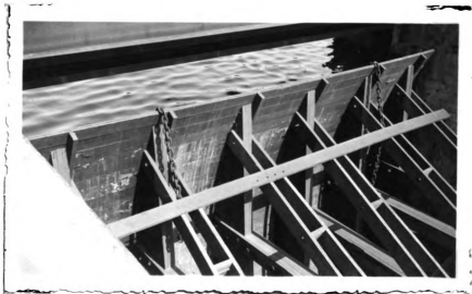
A close-up of one of the above gates. Note the light wood construction, making the gate adaptable to the principle of Part IV of this paper.
