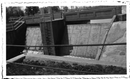
Downstream view of the "Lang" bear trap gates at the Geddes Plant of the Detroit Edison Company. Part of an emergency spillway is shown at the right.
