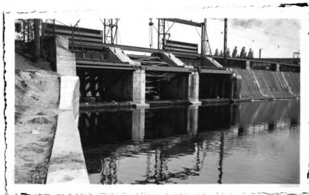
General view of Tainter gates at Moores Park Plant in Lansing, Michigan.
