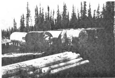
Figure 39. Insulated Water Pipe and Fuel Tanks.
