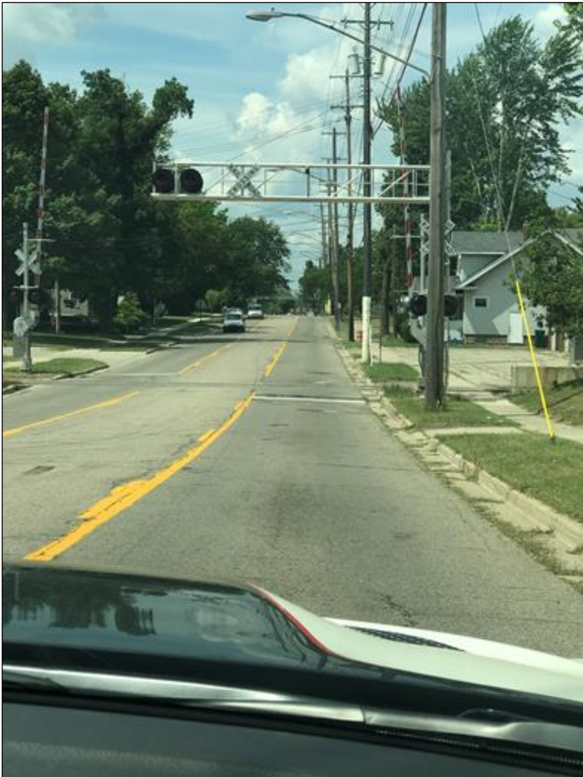
Figure 2.10 This picture is showing the bike corridor interacted with railroad along Mt. Hope Rd. in the Lansing area. As a bikeway, the portion of the road is functioned as Shared Roadway, where cyclists can share the right side of the road with automobiles. However, when the traffic is stopped by the incoming trains, there is no suitable location for cyclists to wait. Also, there is also no appropriate signage for bicycle orientation. The road surface is going to be rough for cyclists when the roadway meets train tracks. Therefore, it is crucial to warn cyclists to slow down beforehand. Copyright © 2017 Yinliang Li, all rights reserved, used by permission.
