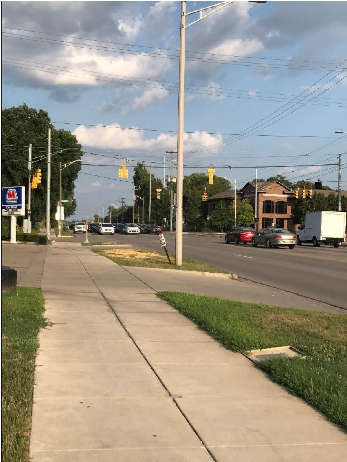
Figure 2.2 The sidewalk in the picture functions as bikeway in the form of Shared Roadway/Sidewalk Bikeways along Grand River Ave. in East Lansing. Cyclists are likely utilizing the sidewalk when there is no designated bikeway. Especially in a higher speed traffic corridor, cyclists often consider traveling on the sidewalk safer. In this case, cyclists are sharing the sidewalk space and traffic rules with pedestrians. However, similar to pedestrians, cyclists riding on the sidewalk still face the potentials danger causing by turning automobiles. Copyright © 2017 Yinliang Li, all rights reserved, used by permission.
