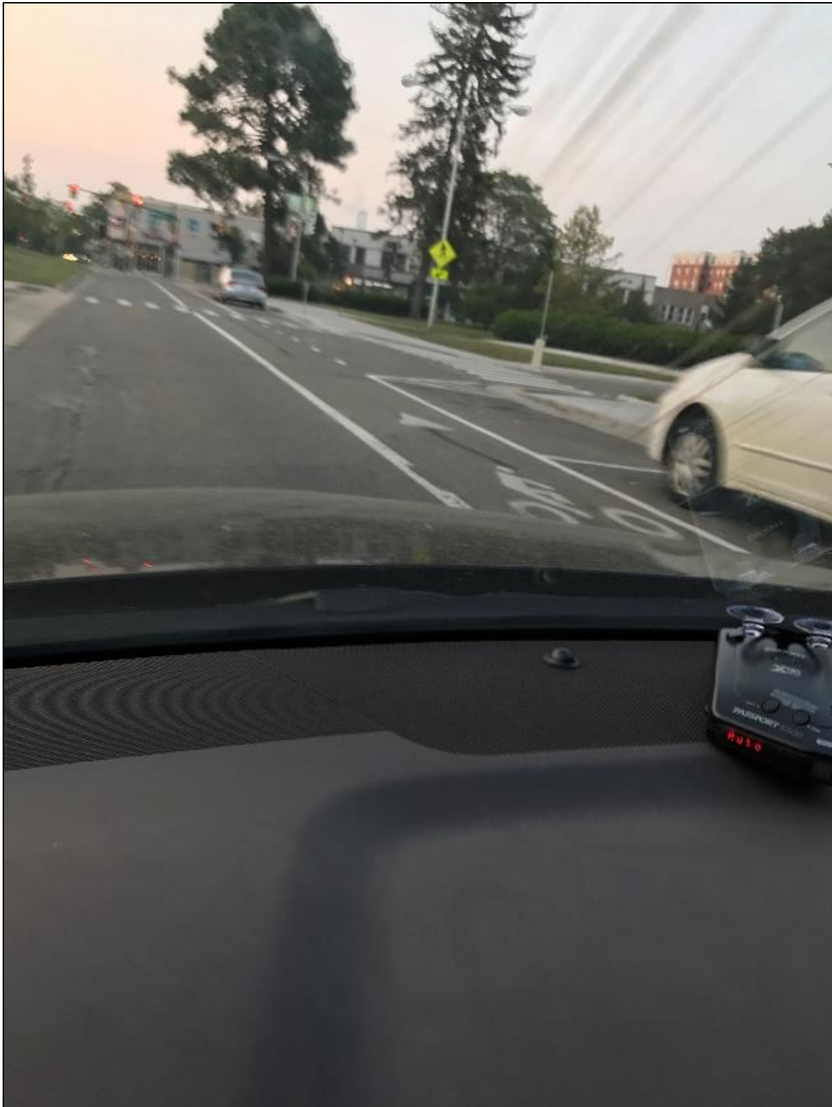
Figure 2.3 The picture is the bike lane (with symbols and marking) on Abbot. Rd in East Lansing. This bike lane is designated for cyclists, and it is installed between a roadway and a strip of parallel parking spaces. From the observations, the narrow width of the bike lane limits the usage of this bikeway. There are also potentials that cyclists encounter with automobiles as well as people exiting from parked cars. On the other hand, this bike lane intersects with MSU Union drop-off area, which is a busy location that might interrupt the continuity of riding. Copyright © 2017 Yinliang Li, all rights reserved, used by permission.
