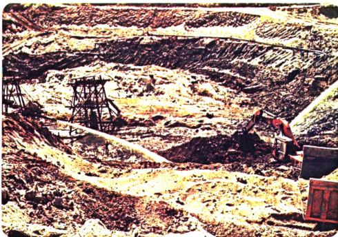
Exhibit 2 - Breaking the earth by using both Excavator and Water-pump. This process is applicable in the gravelpump and other opencast mining methods.
