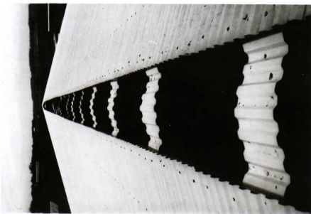
Figure A.4 Flashing at the open ridge-- Barn I
