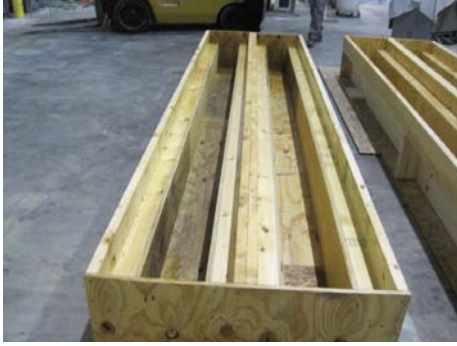
(a) Preparation of wood forms
