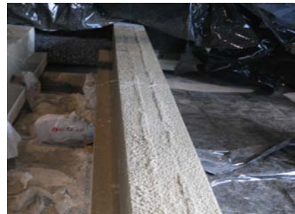
(b) Spray a dash coat layer
