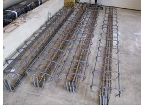
(b) Assembling reinforcement cage
