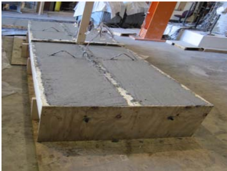
(c) Casting of concrete
