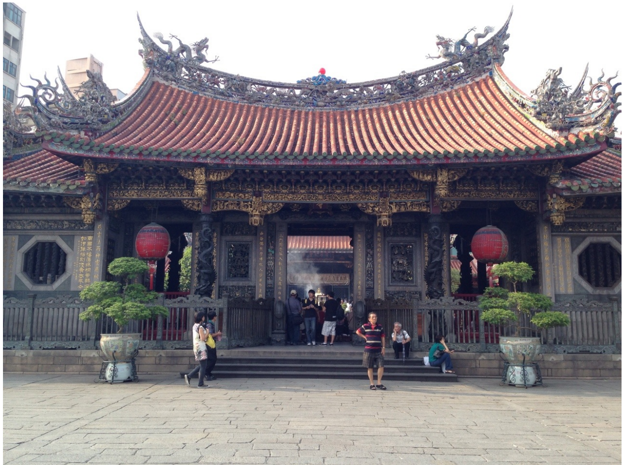
Figure 1.6 Longshan Temple, Taipei, Taiwan (Copyright © 2013 Li-Yueh Chu, all rights reserved, used by permission)
