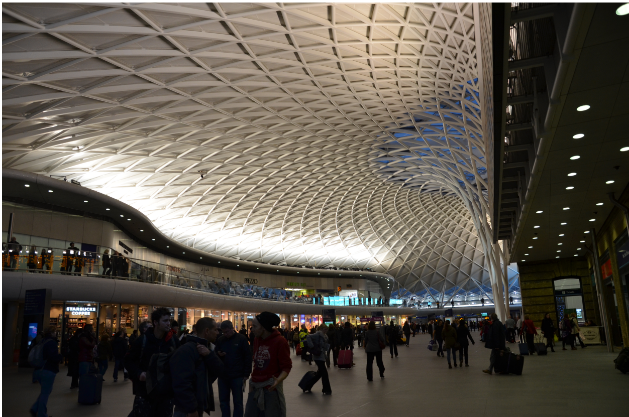
Figure 1.4 King's Cross Station, London, UK (Copyright © 2013 Wan-Chu Lin, all rights reserved, used by permission)
