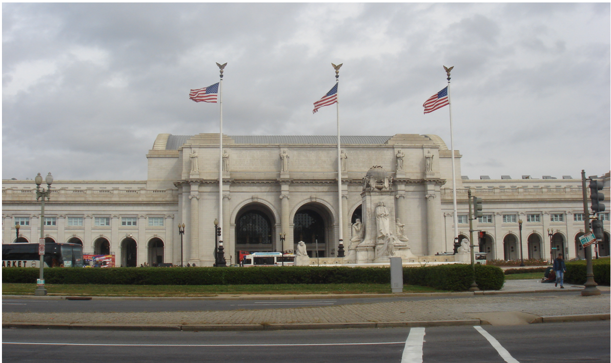
Figure 1.7 Washington DC Train Station, USA (Copyright © 2008 Wan-Chu Lin, all rights reserved, used by permission)
