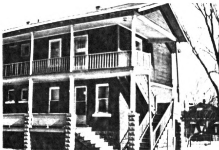
Figure 60.--Canadian French Style House (Poteaux-sur-sol).
