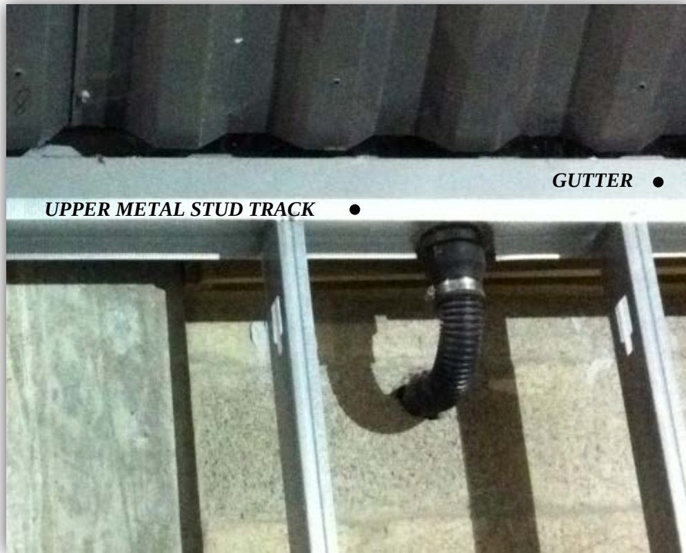
Figure 4.20 – Upper Metal Stud Track and Gutter – Construction Outcome
