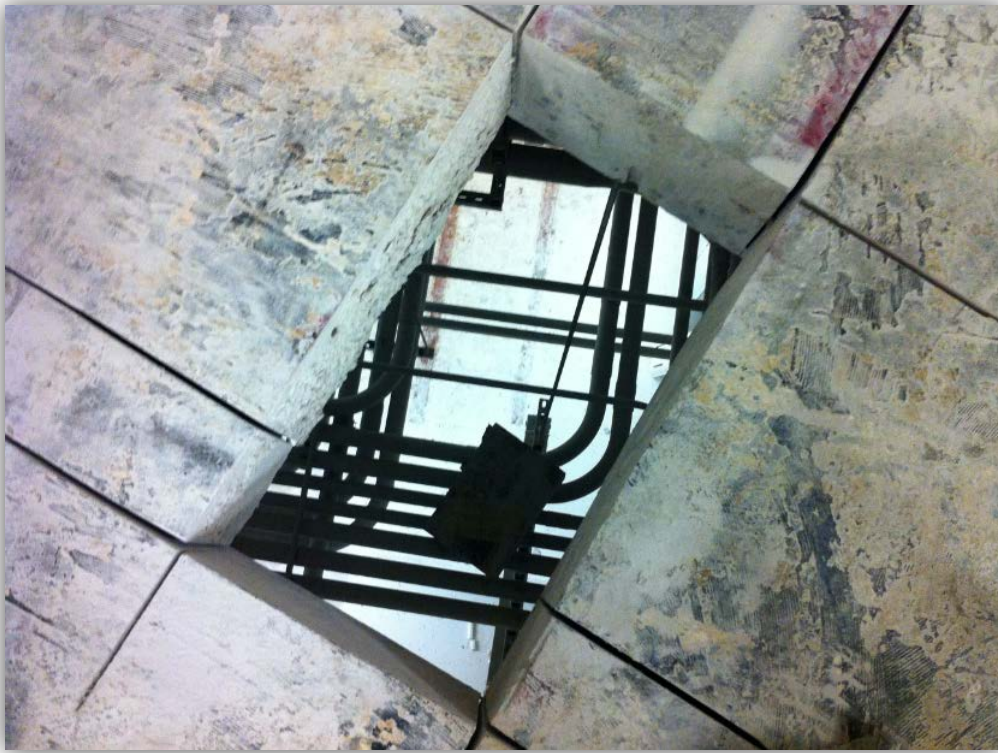
Figure 4.21 – Concrete Utility Trench – Demolition Outcome
