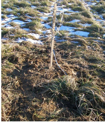
Figure 3-19 The installed site after installation. Two tube, clear and blue, for water sampling and a cable for signal transmission come out of the draingage.
