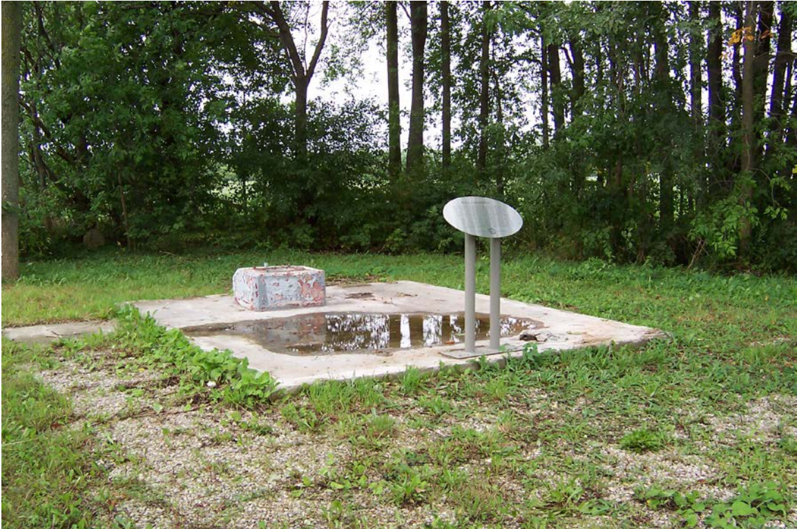
Figure 18: Well 5 after it was sealed. Well 5 in Walkerton was sealed after the E.coli contamination and a plaque placed there commemorating the event. The Biesenthal cattle farm is just beyond the trees. In the spring, this area floods, turning it into a pond where ducks swim (interviews).
