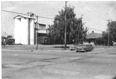
(15) St. Johns. Railroad station (freight only) and a grain elevator. There is a relatively large-scale factory behind the station.
