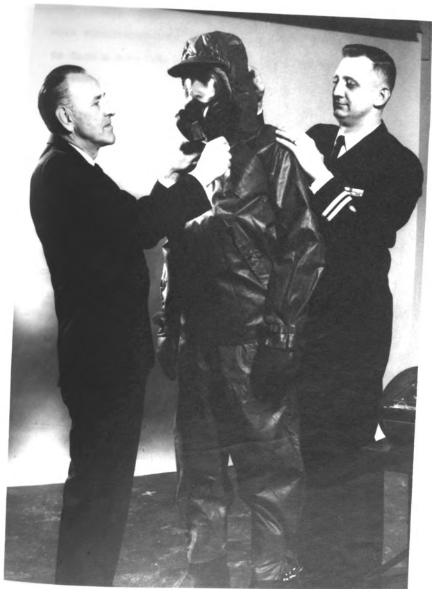
Figure 6. Impermeable, unventilated, protective garment.
