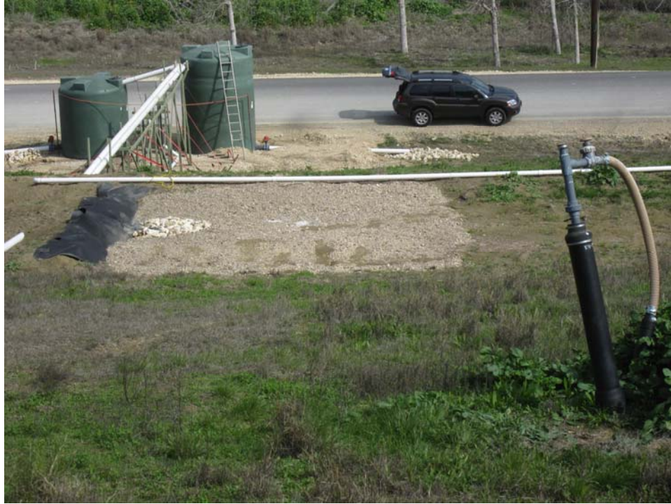
Figure 1-3. Runoff collector pad for lower catchment
