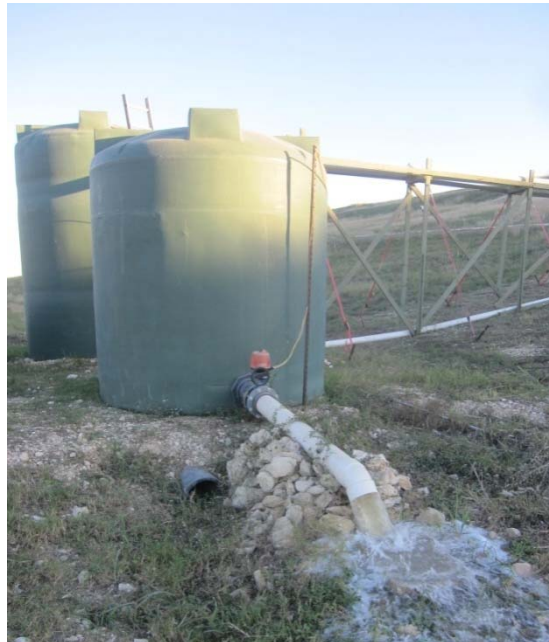
Figure 1-4. Actuator controlled valve draining upper catchment AST
