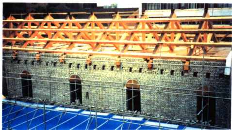
Figure 74. Wooden truss frames, Cathedral construction site. Photo by Daewoo Construction Co.
