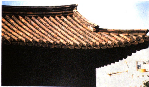
Figure 21. Korea's traditional roofing materials and eaves. Photo by Pilhoon Jin & author.
