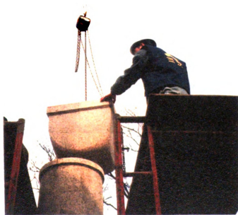
Figure 72. Constructing a column, Cathedral construction site. Photo by Daewoo Construction Co.
