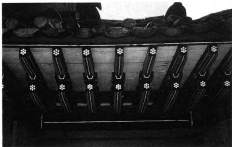
Figure 49. Exposed rafter tails of a traditional Korean house. Photo by Pilhoon Jin & author.
