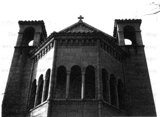
Figure 28. Thin engaged corner columns and modillions on the cornice, apse. Photo by Pilhoon Jin & author.
