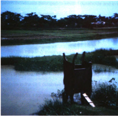
Figure 3.5 Hanging latrine on a small canal.
