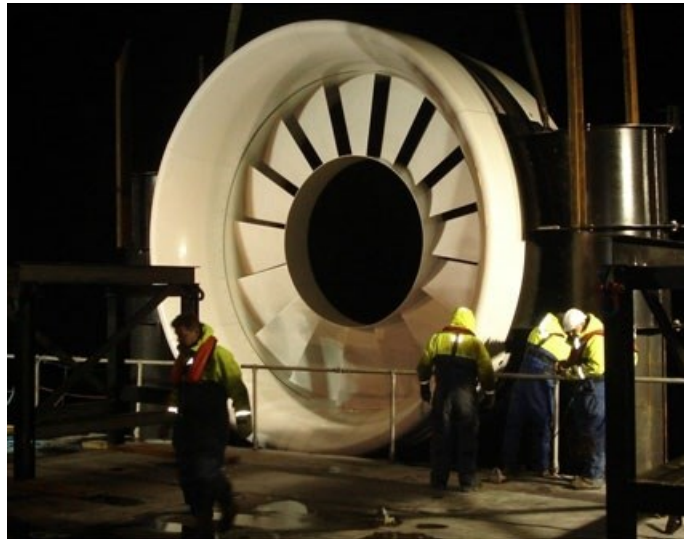
Figure 6.1 Open Hydro Open-Centre Turbine
